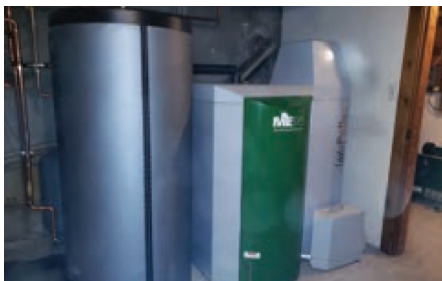
Biomass heating indoor unit
