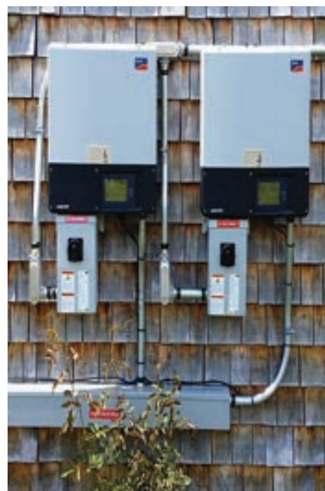
Inverters installed outside of residence
