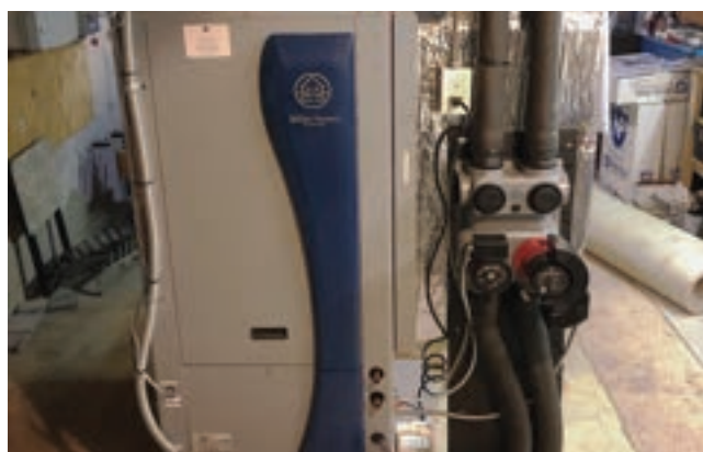
Ground-source heat pump indoor unit
