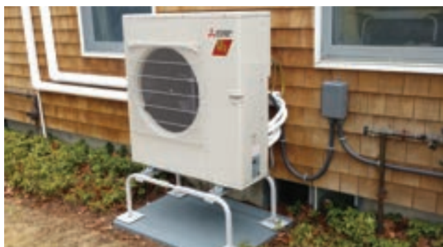
Air source heat pump external unit
