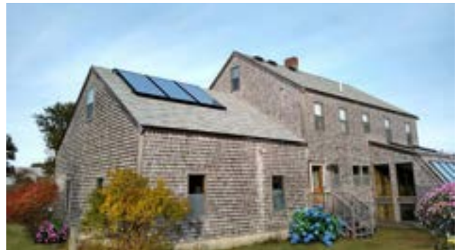
Solar hot water system
